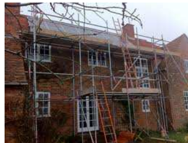
Local scaffold companies x 5
